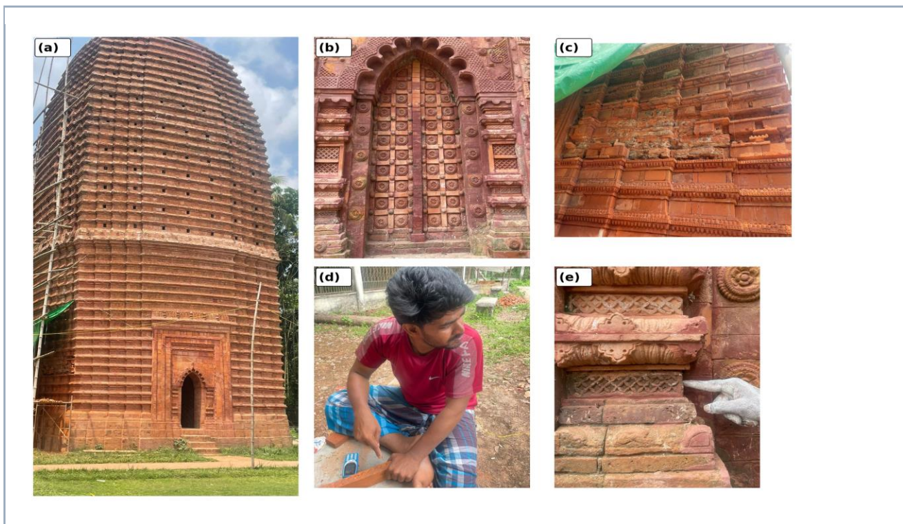
Figure 2: Kodla Moth during ongoing conservation: (a) overall exterior and scaffolded work zone; (b) surviving ornmented entrance; (c) major local loss exposing irregular masonry; (d) artisan handling a newly produced patterned terracotta element; and (e) visual relationship between weathered historic fabric and newly worked areas. Photographs by the author, 2 April 2026.
